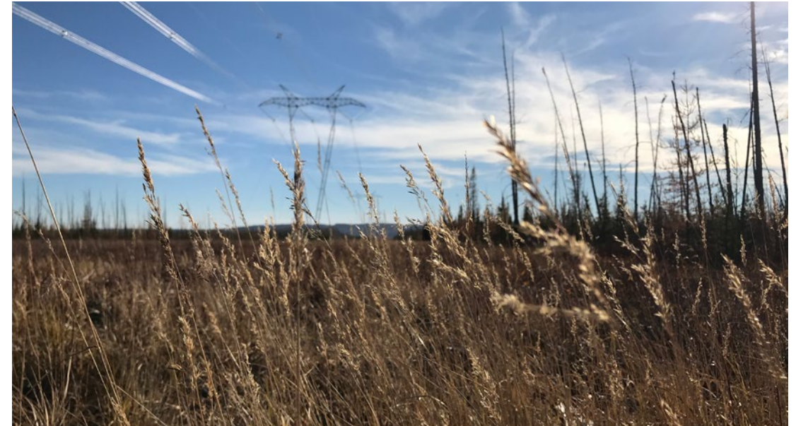
Land is reclaimed along Alberta PowerLine's (APL) Fort McMurray West 500-kilovolt transmission line.
