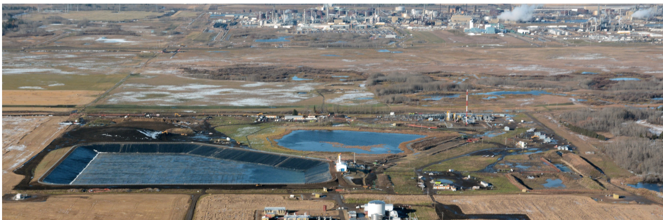
ATCO Heartland NGL storage facility, Fort Saskatchewan, Alberta
