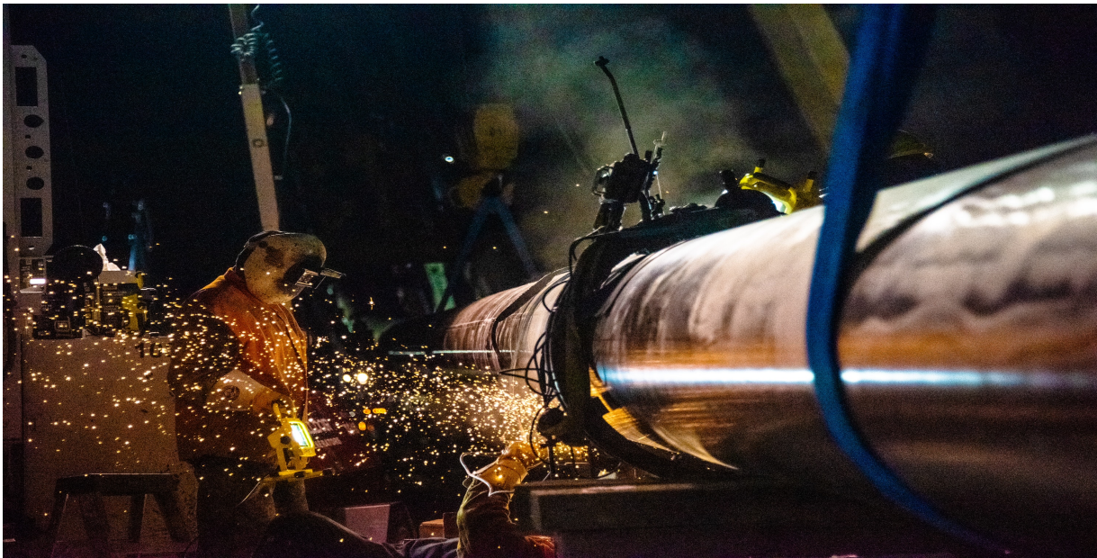
Pembina-Keephills transmission pipeline construction, near Wabamun Lake, Alberta
