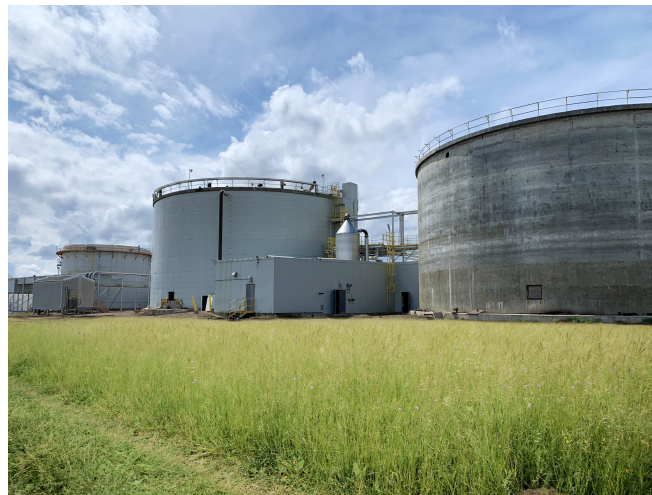
Two Hills Renewable Natural Gas (RNG) Facility - Vegreville, AB
