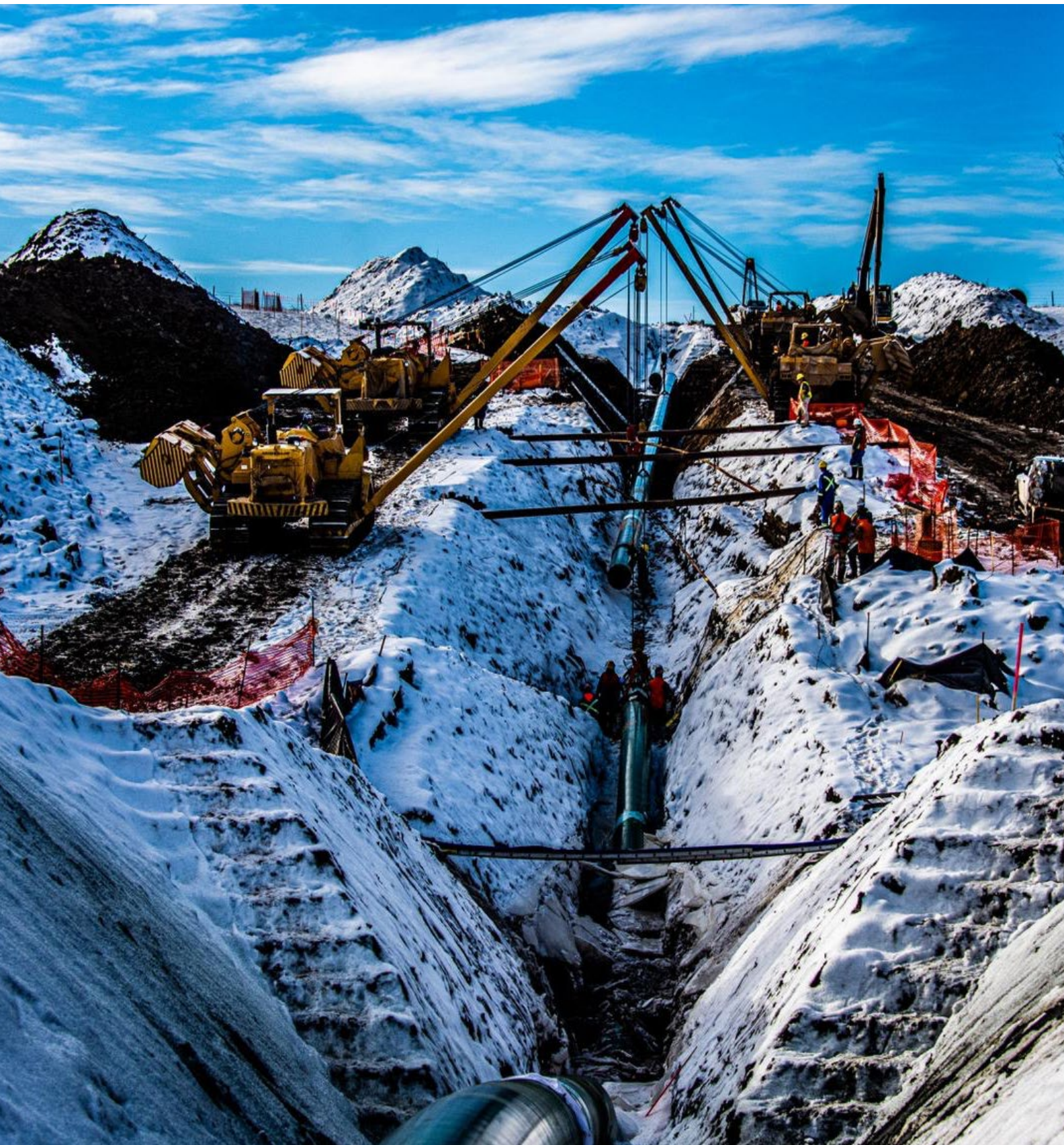
Pembina-Keephills Transmission Line construction.
