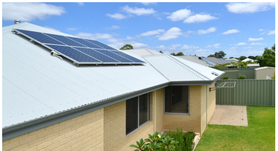
Australia residential rooftop solar panels.
