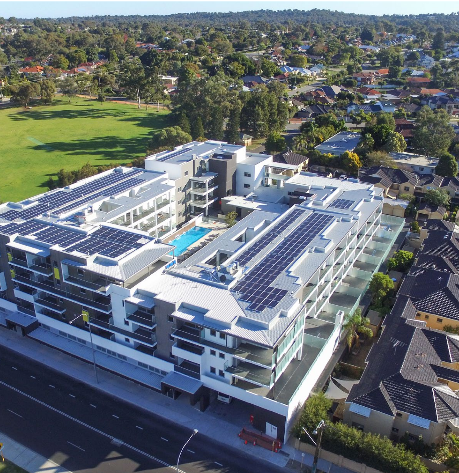
The Park Avenue building in Churchlands, Western Australia, utilizes rooftop solar panels and other energy-efficient designs to provide building residents with a sustainable source of energy.
