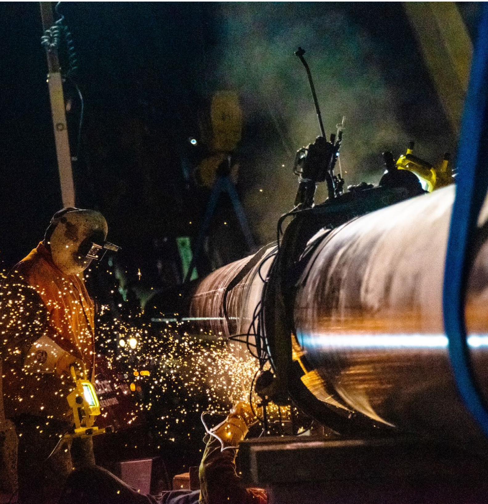
Pembina-Keeyhill Transmission Line construction.
