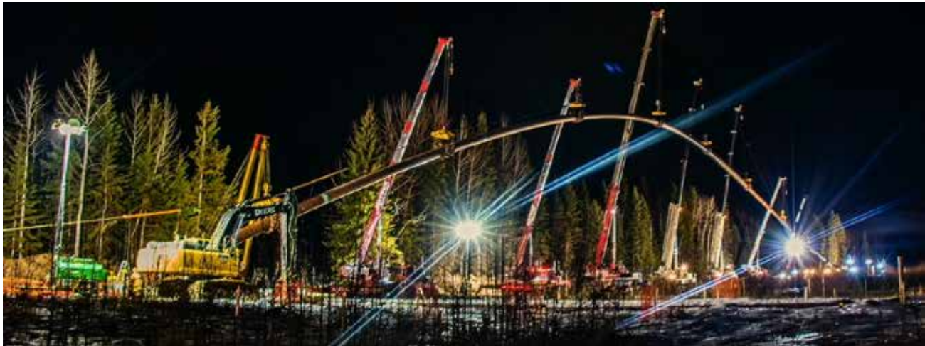
Pembina-Keephills transmission pipeline construction, near Wabamun Lake, Alberta
