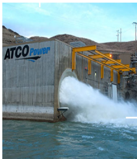
Oldman River Hydroelectric Plant
