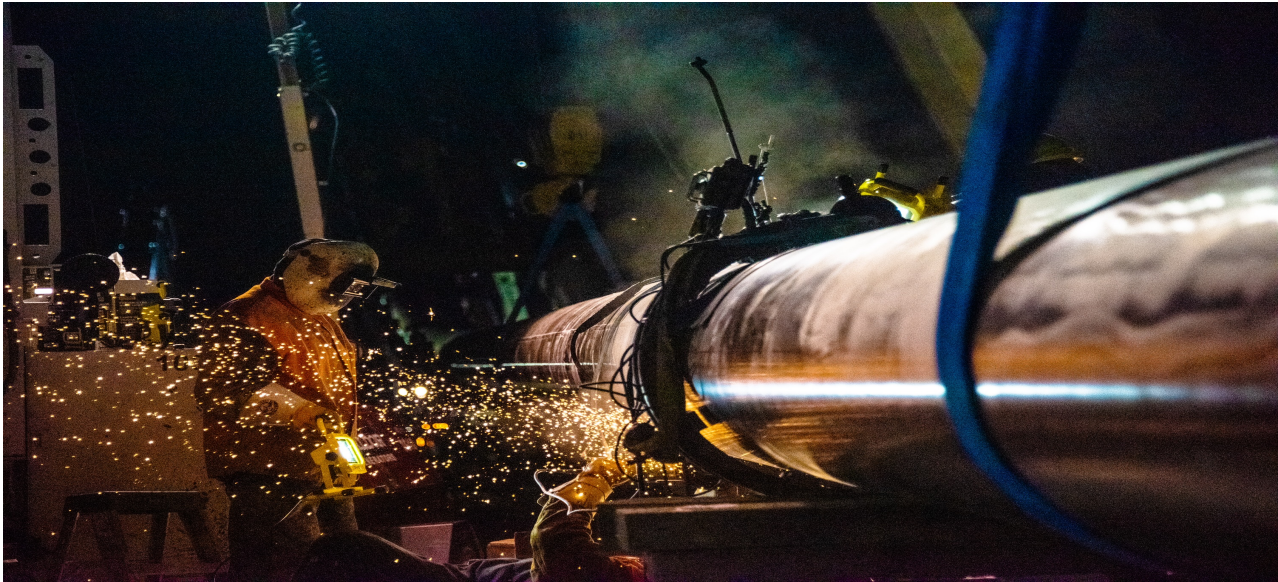
Pembina-Kepphills transmission pipeline construction, near Wabamun Lake, Alberta
