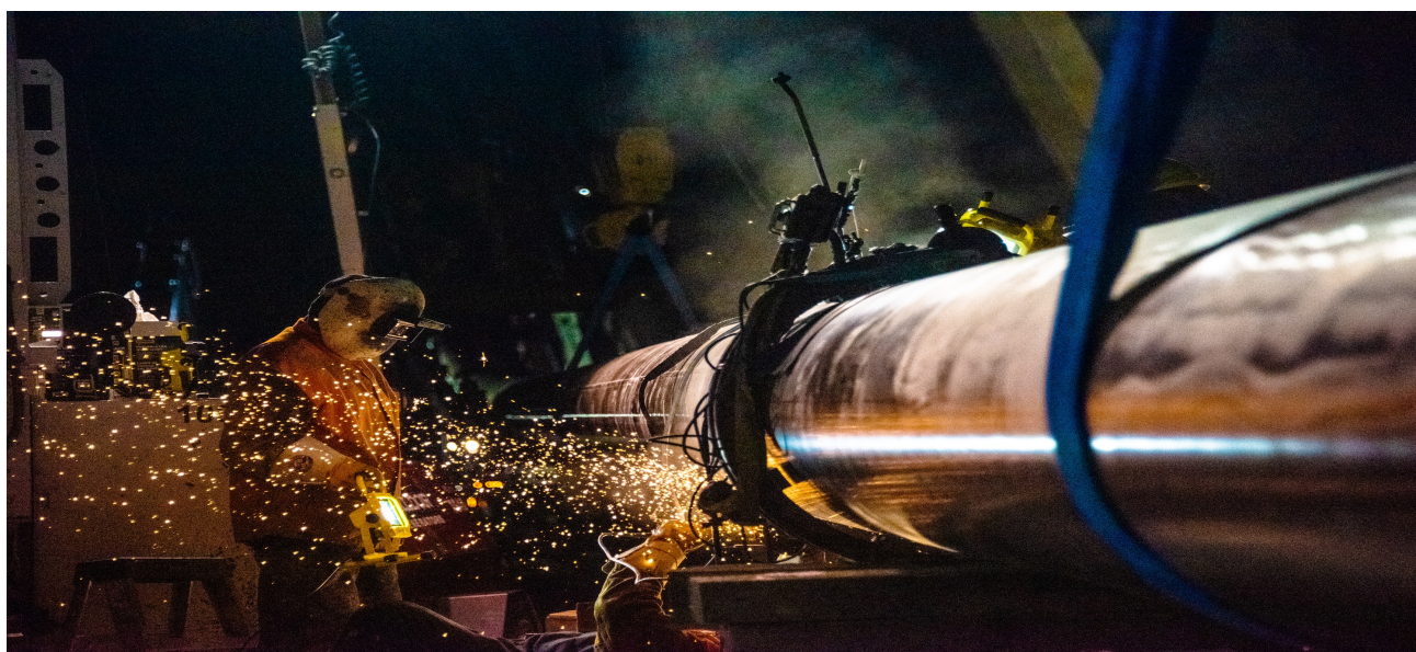
Pembina-Keephills transmission pipeline construction, near Wabamun Lake, Alberta
