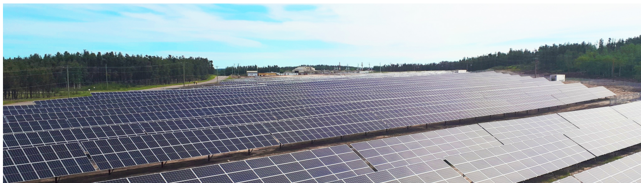
Fort Chipewyan Solar Project, Fort Chipewyan, Alberta
