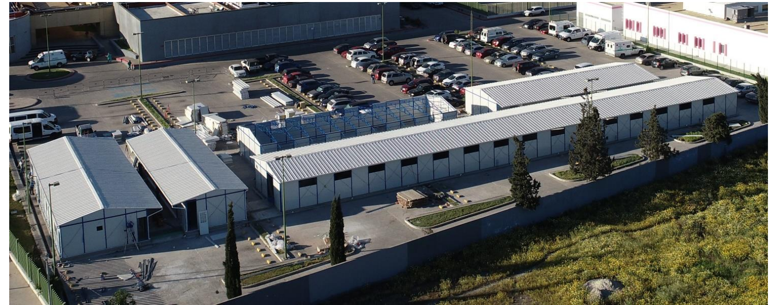
Modular Hospital Facility, Tijuana, MX
